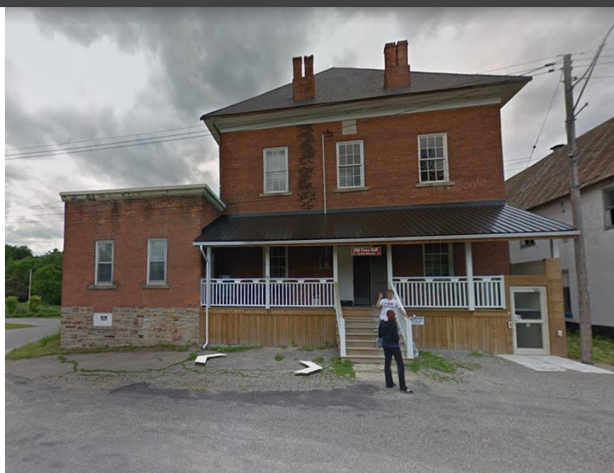
Figure 3 Building A – Old Town Hall
